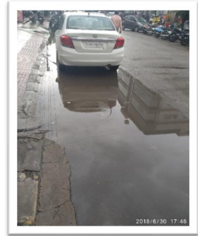
Exhibit 4.8: Photographs showing unscientific construction of roads/drains – absence of proper gradient/alignment
